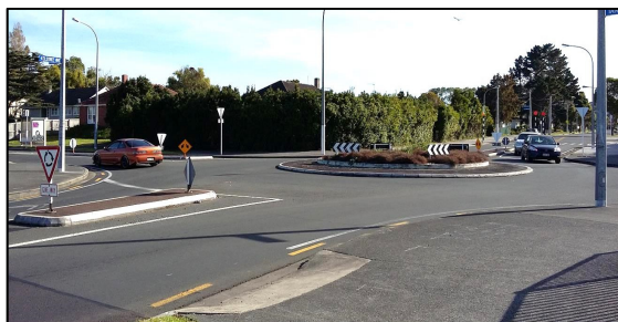
1) Taniwha Street/Elstree Avenue Roundabout
