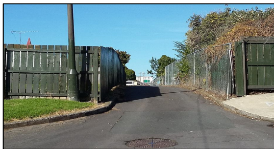
3) Existing Pump Station Access (Maybury Street)
