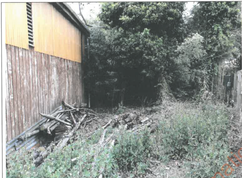
5. View behind the current fire depot
