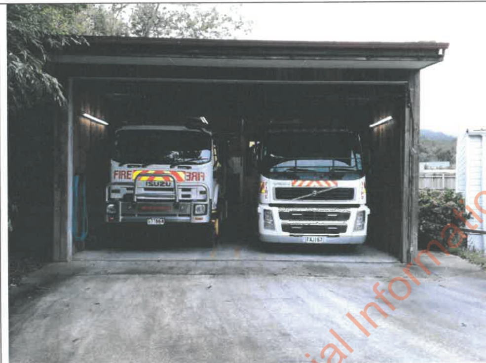
1. Building can barely fit their appliance and tanker
