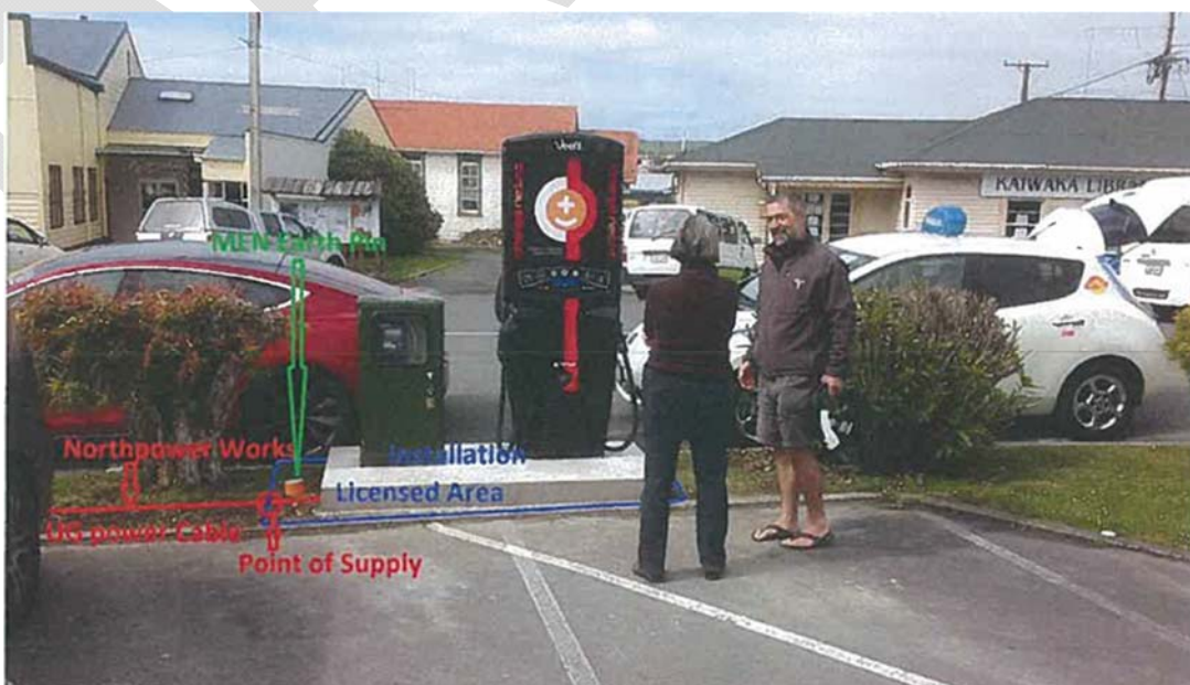
Figure 1: photo of road side EV charger (provided by Northpower, the electricity distributor in Northland)
