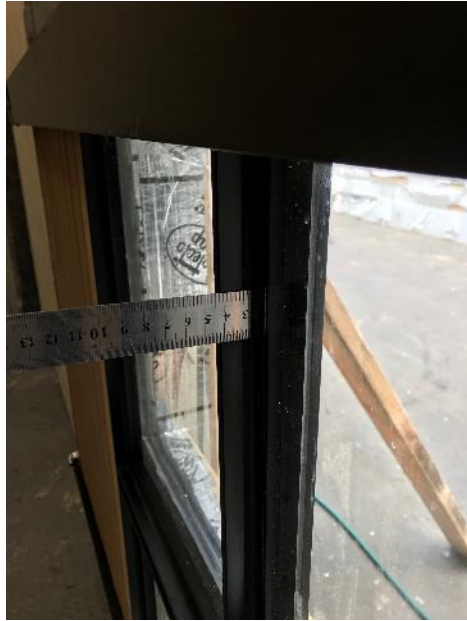
Figure 3 – Pane 1, Left Jamb Seal
