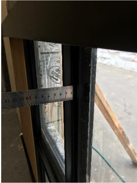
Figure 3 – Pane 1, Left Jamb Seal
