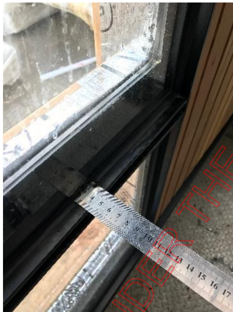
Figure 5 – Pane 1, Sill Seal
