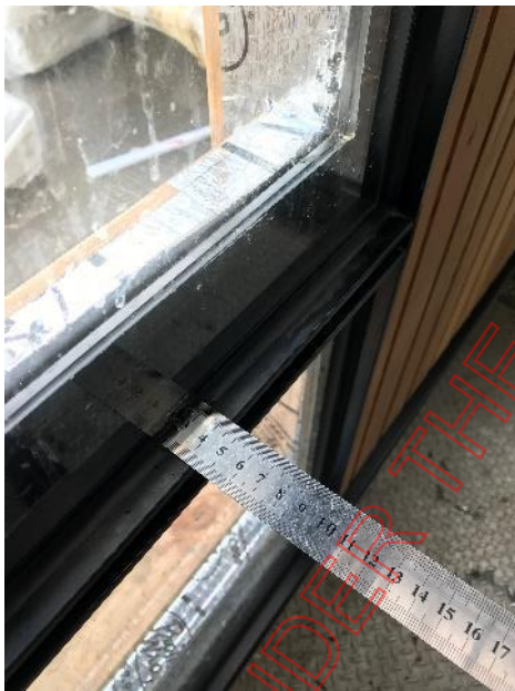
Figure 5 – Pane 1, Sill Seal
