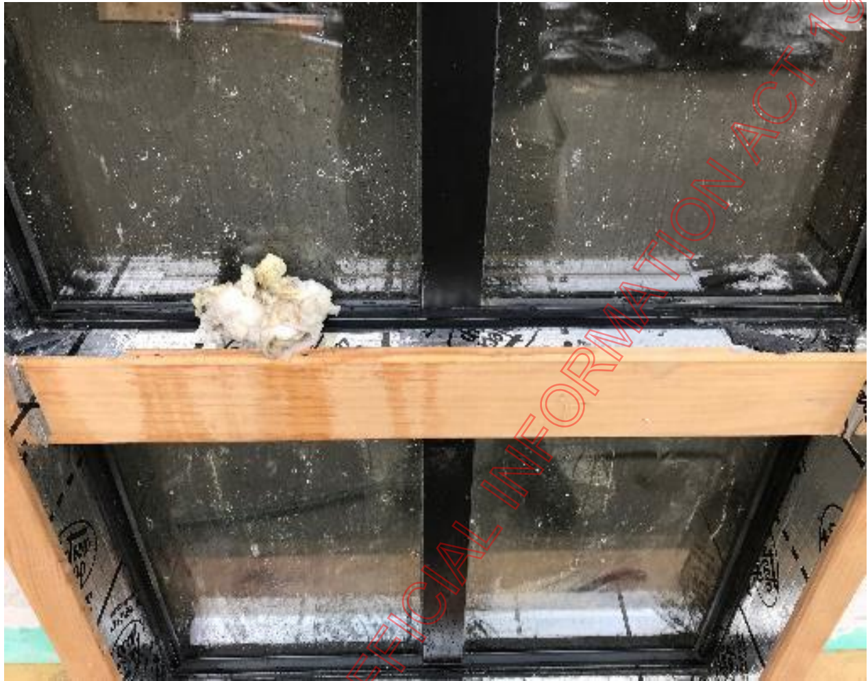
Figure 7 – Panes 1 & 2, with Interior Seals removed, during testing
