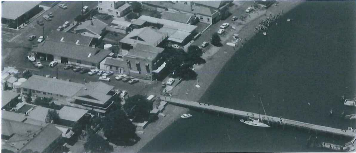
Plate 12: Detail of Plate 11, showing the absence of the buildings at the shore end of the wharf (Turnbull Library)
