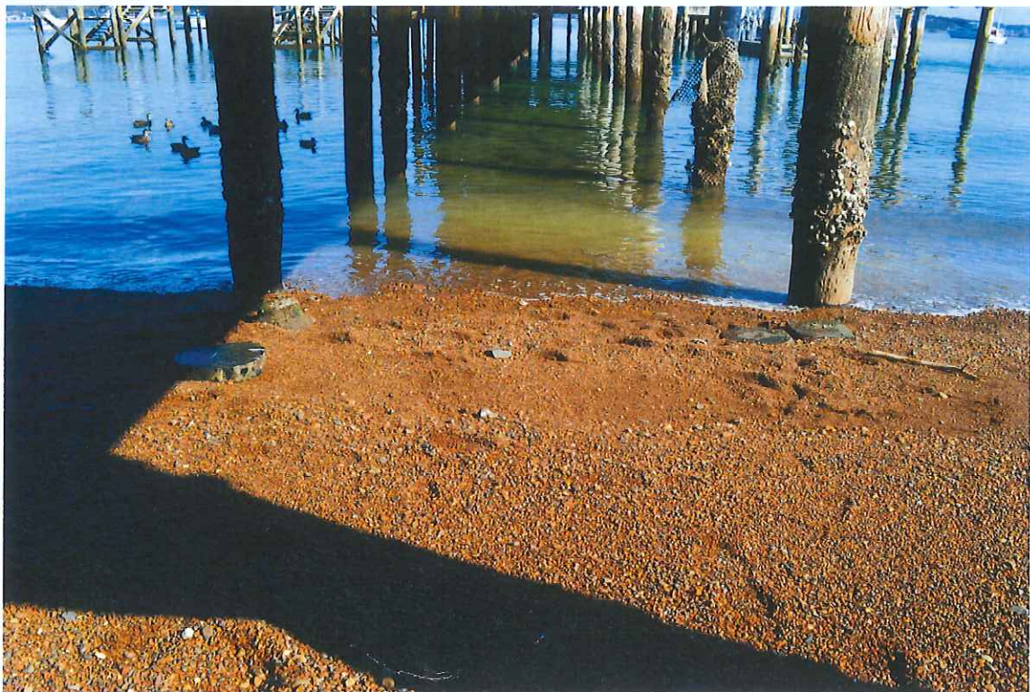
Plate 15: The remaining piles visible below the current Russell wharf
