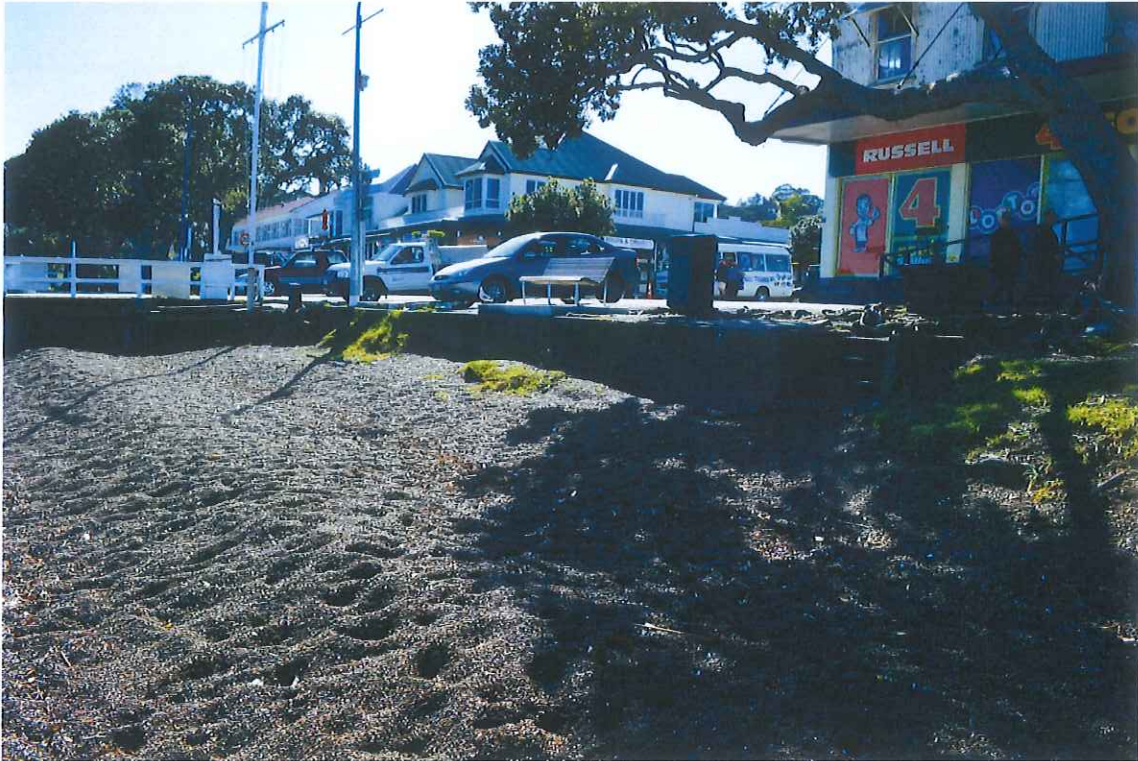
Plate 13: The current concrete retaining wall located to the immediate south of the Russell wharf
