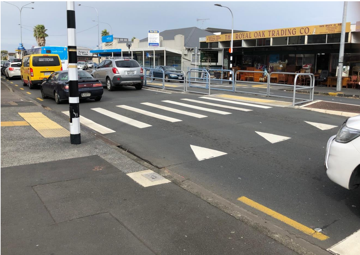
Figure 2 Vertical deflection at raised pedestrian crossing of Mount Albert Road
