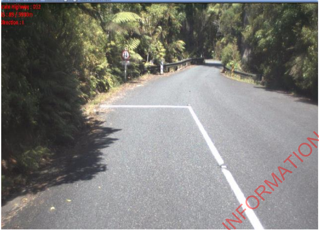
View looking north toward the bridge
