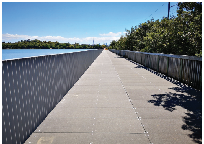
Section 3 new decking
