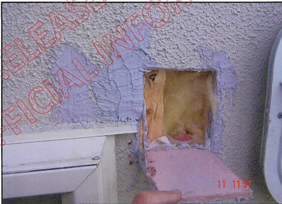
Reopening of existing previous cut out
