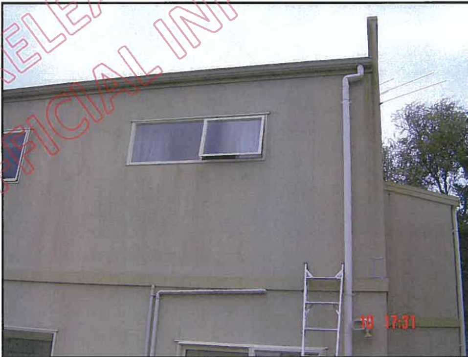
General view-part rear elevation (west) unit E
