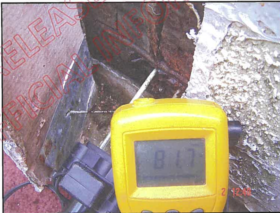
Cut out and high probe reading; south wall at base showing advanced fungal decay to frame and bottom plate
