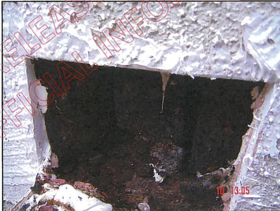
Close up of photograph 5d 116: showing total decay to bottom plate and frame
