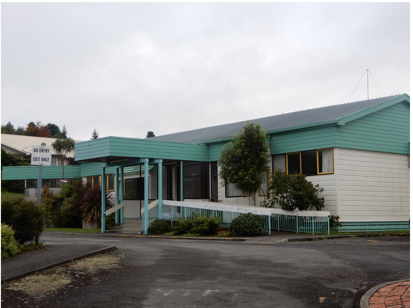
Taihape Hospital, Main Maternity Building Interior Asbestos Assessment.
