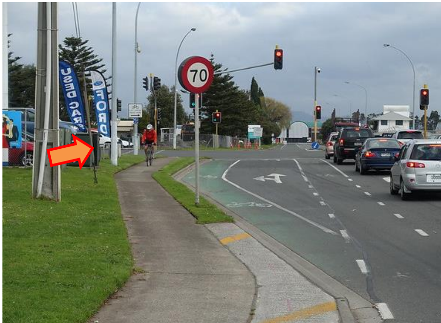
Figure 10: Strainer wire (highlighted)
