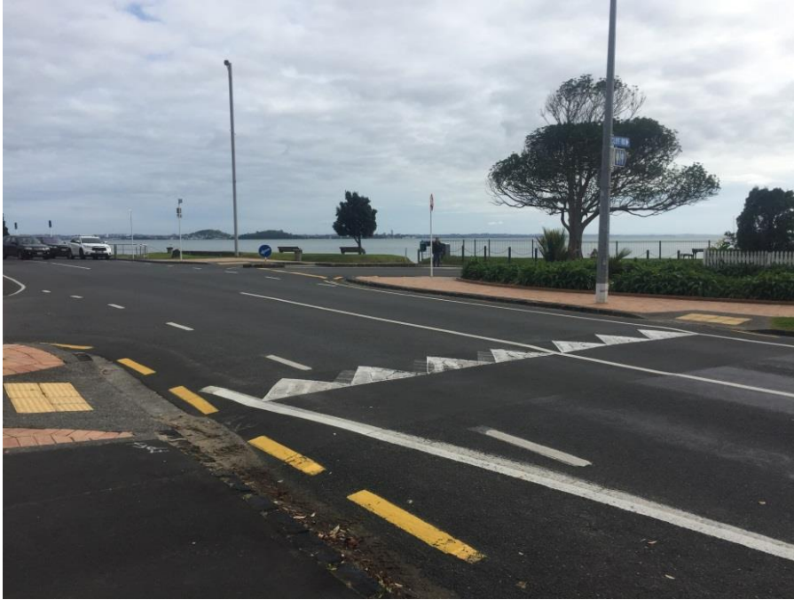
Figure 10: Kerb crossing with no formalised crossing facilities
