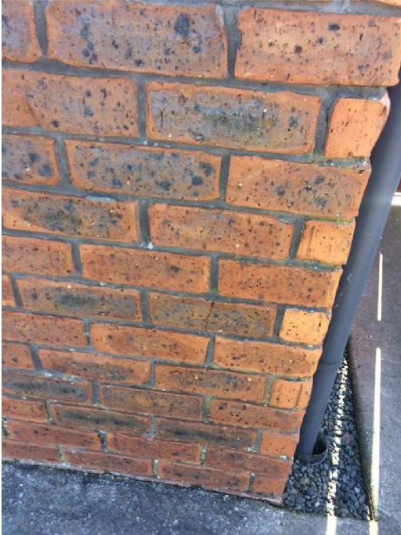
Figure 4 : South west Garage corner
