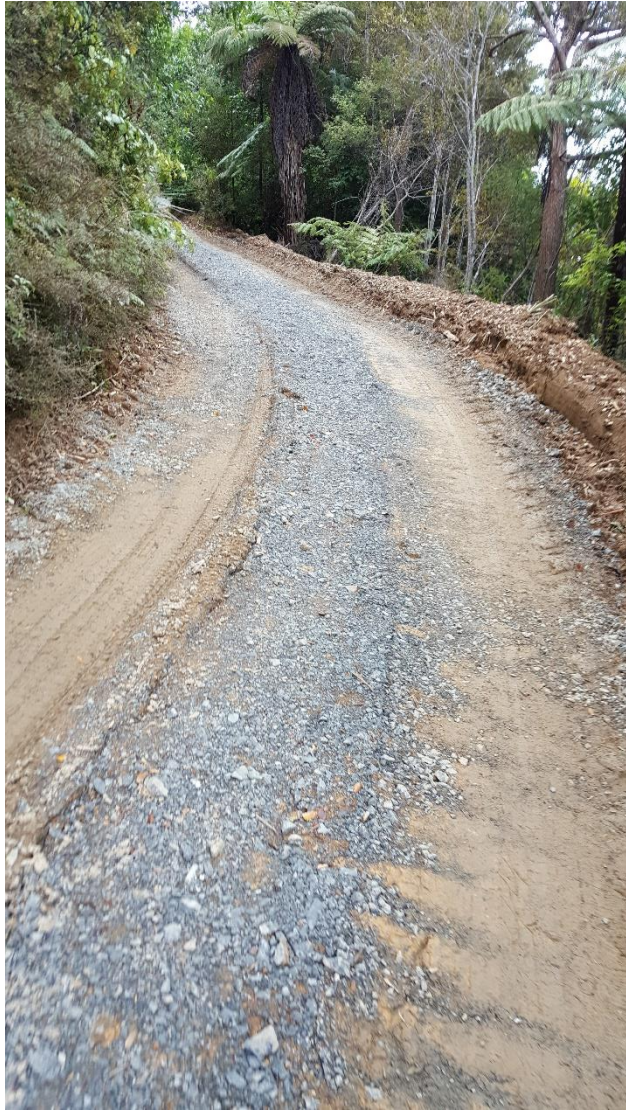
Example of margins of the track showing mud exposed by recent vehicle movement
