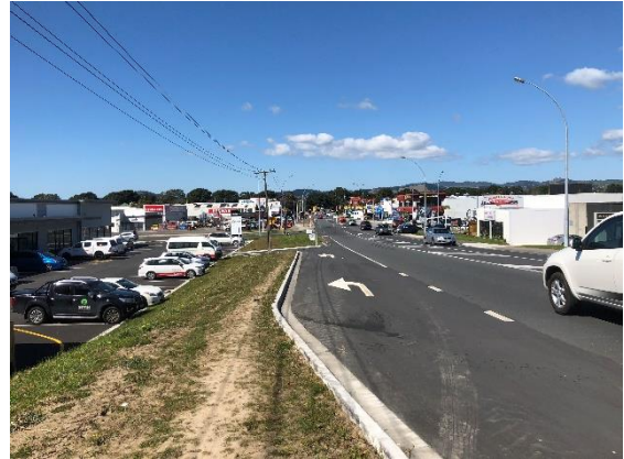
Photograph 6: Existing left turn slip lane to retail outlets on the northwest corner of Burrows Street intersection.
