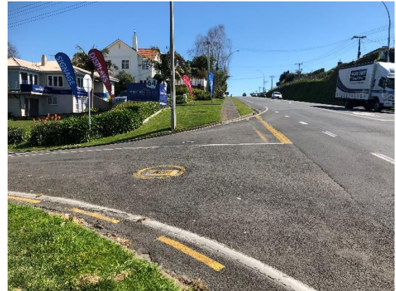
Photograph 4: Existing steep berm on southwest side of Scantlebury Street
