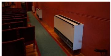
Heating in the auditorium is provided by water-heated radiators mounted on the internal walls; the water in turn is heated by a diesel-fired boiler, which is housed in a specific building adjoining the loading dock. The heated air rises to the upstairs seating, from where it is dispersed by vent chutes in the circle area ceiling, and recirculated by fans back into the rear stalls area.
