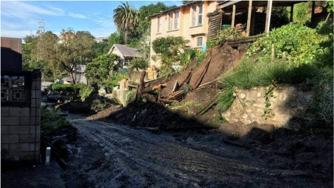
Figure 87: Roading damage on Brewster Rd, Napier Hill.
