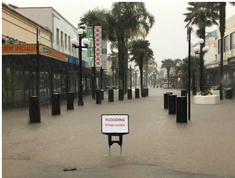
Figure 13: Emerson Street flooding, 9th November 2020
