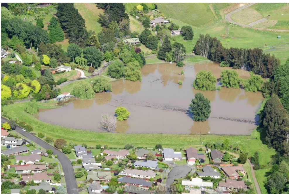
Figure 28: O’Dowd Dam post flood, 9am 10 th November (Photo credit – Peter Scott).
