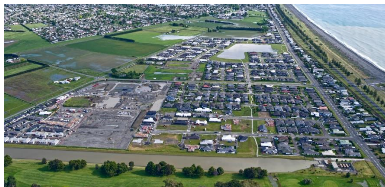
Figure 75: Te Awa subdivision showing detention pond, 8am 10 th November (Photo Credit – Peter Scott)
