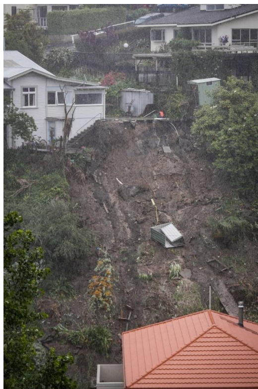
A number of slips have been reported across Napier. Photo / Warren Buckland
