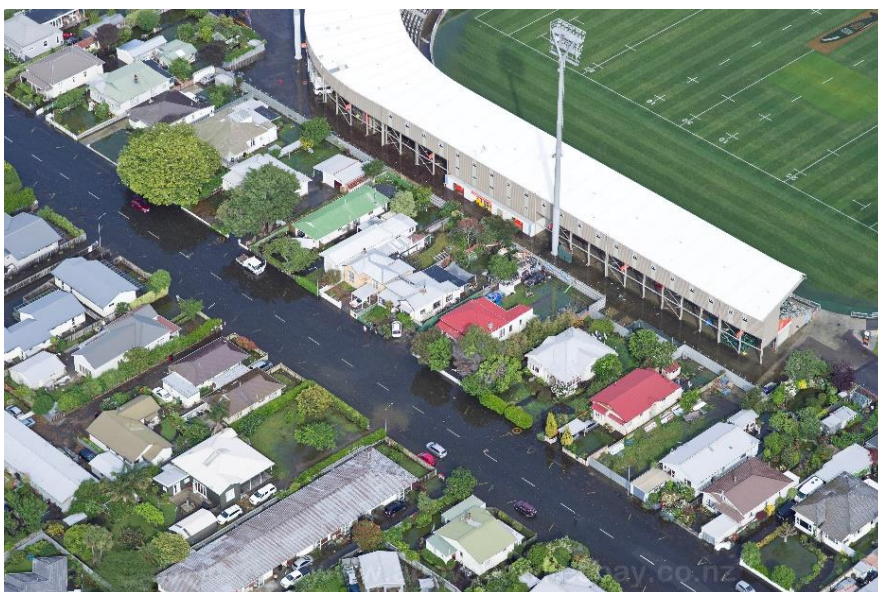
Figure 12: Latham Street and McLean Park flooding, 10th November 2020 (Photo credit – Peter Scott)
