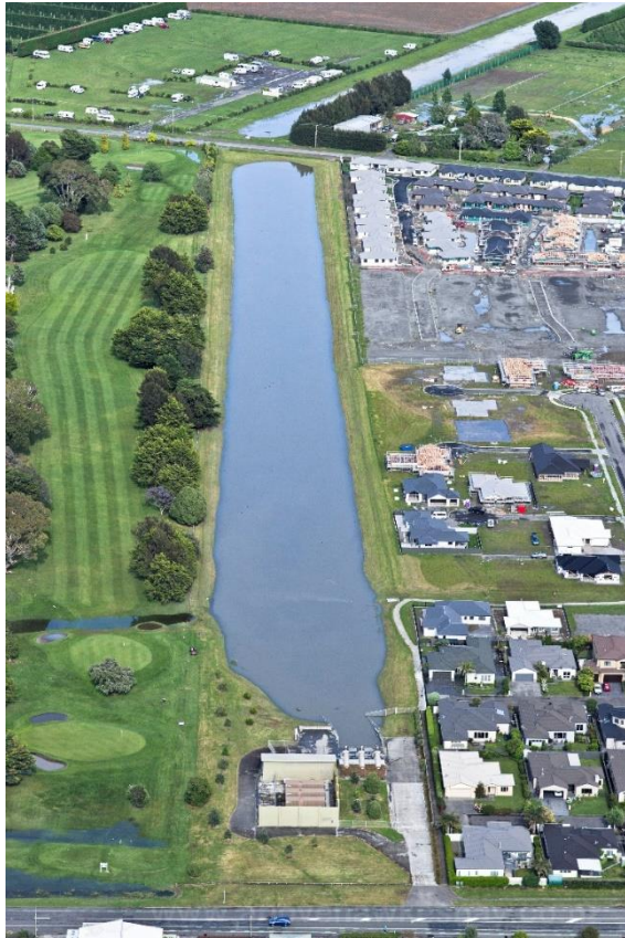
Figure 18: Cross Country pumping station, 10th November 2020 (Photo credit – Peter Scott).
