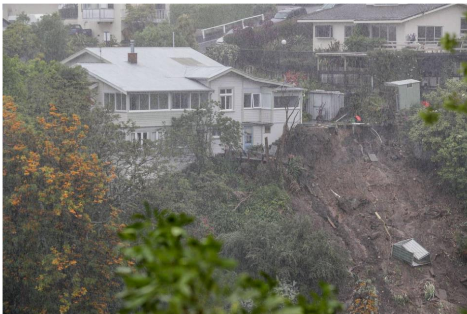
A large landslide swept away a structure on Hospital Hill, near Havelock Rd. Photo / Warren Buckland
