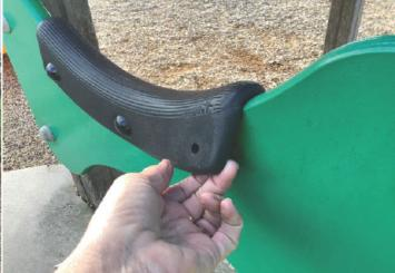
Finding: Cover is loose Action: Secure all loose fixings
