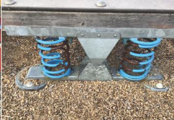
**Finding:** The paintwork on the spring has been damaged or **Action:** Treat any rusting components and repaint worn exposing the metal underneath which is rusting
