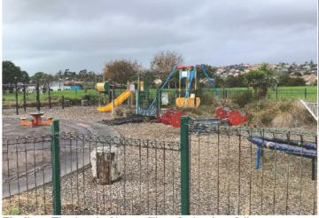
Finding: The level of loose fill surfacing has fallen significantly below the minimum 300mm recommended by NZS 5828:2015 Part 1
