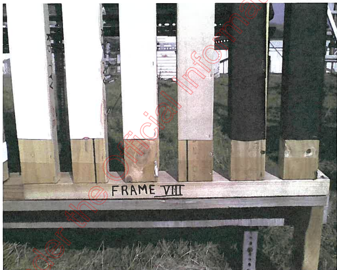
Figure 22. Samples of building wrap weathering in contact with timber treatment chemicals
