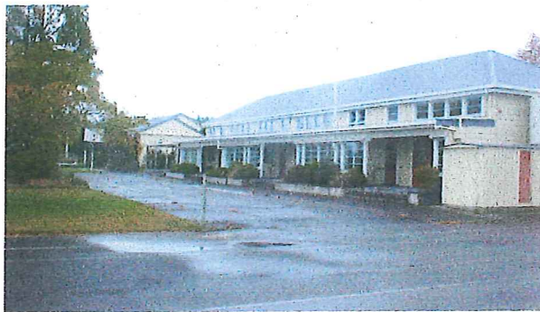
Main class room block with second class room block in background
