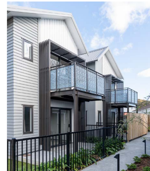
Location: Seddon Street, Naenae, Lower Hutt
