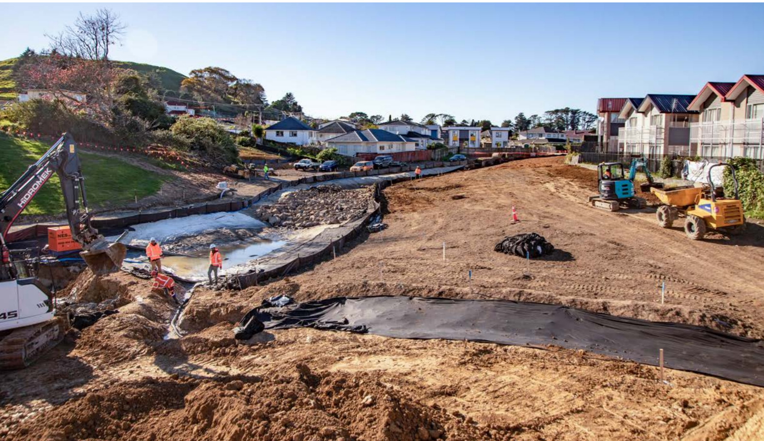
Location: Freeland Reserve earthworks, Mt Roskill, Auckland
