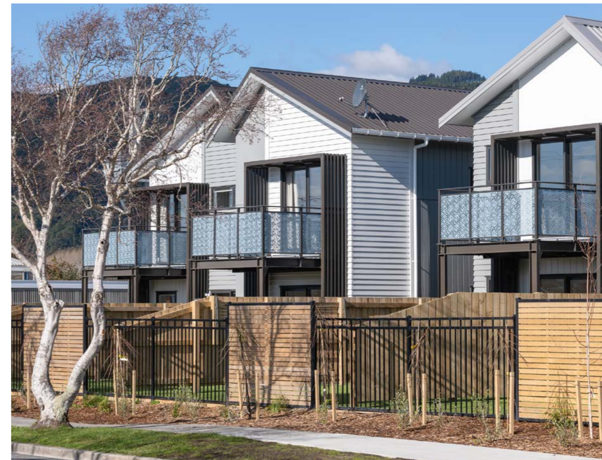
Location: Seddon Street, Naenae, Lower Hutt
