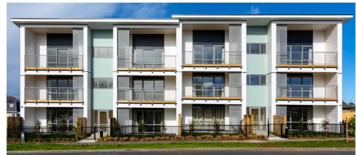
Location: Cambourne Road and Shirley Road, Papatoetoe, Auckland
