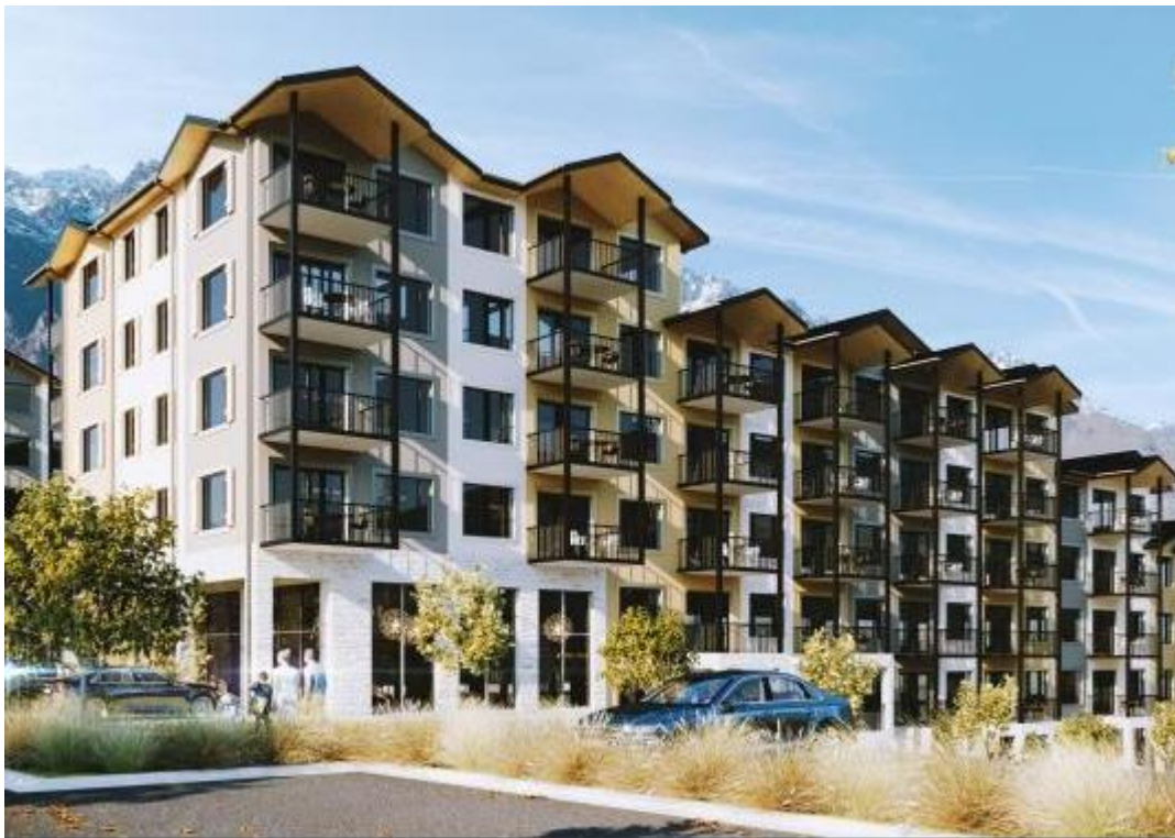
Picture - New assisted housing units through inclusionary zoning in Queenstown
