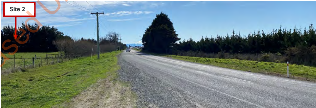
Figure 4.2 Springston Rolleston Road looking north from Site 2 frontage
