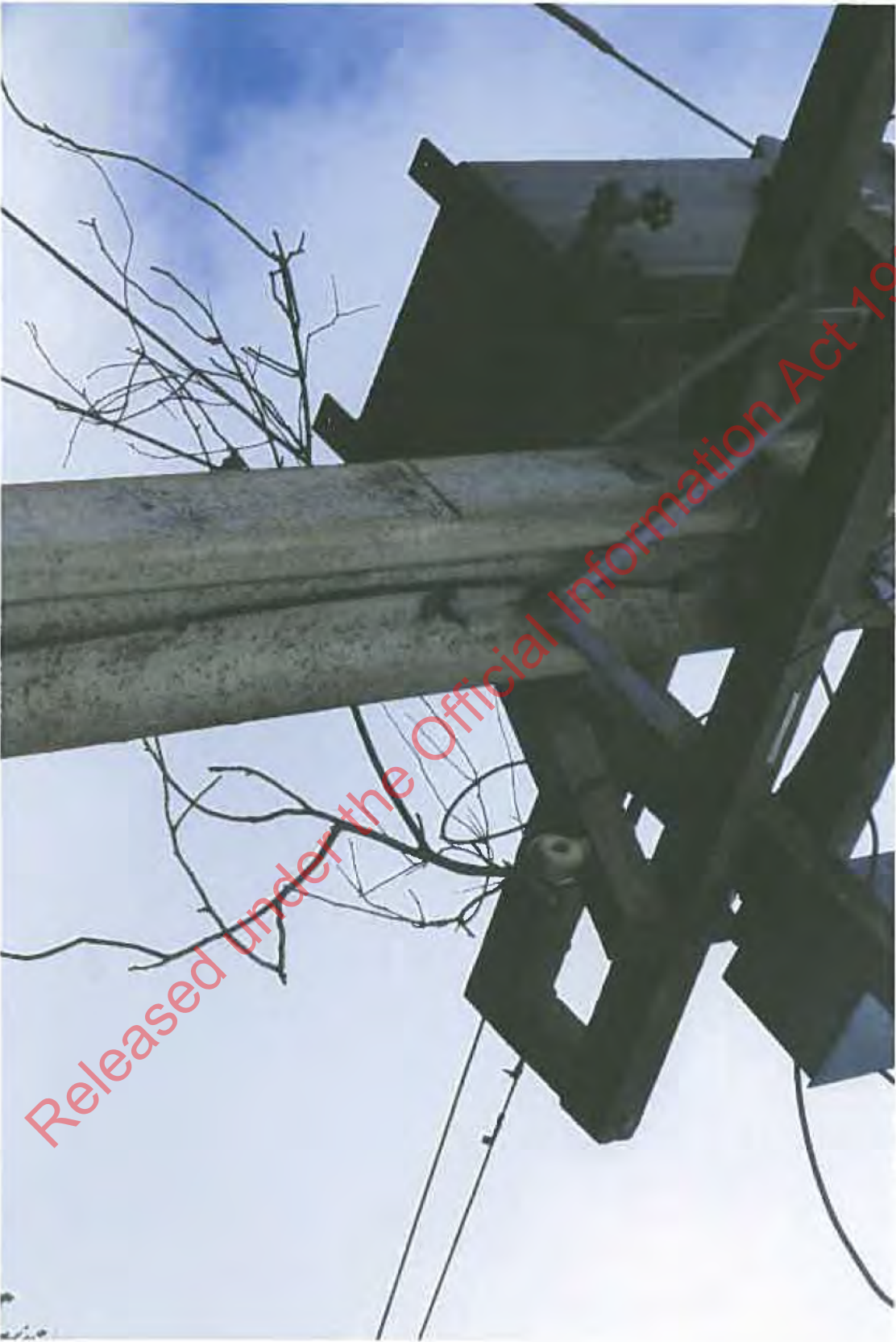
Photos 917 – Approaching the scene, Power pole just prior to 231 Morris road showing branches blown up into the attached telephone line.
