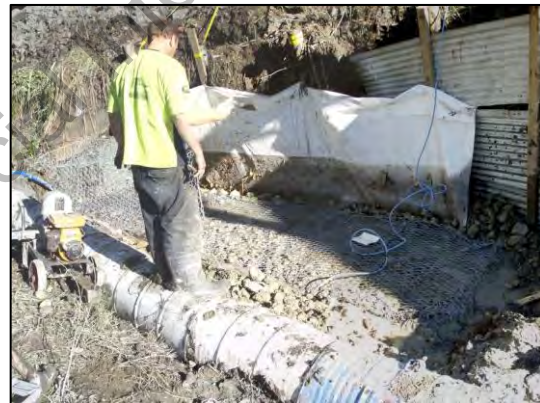
Figure 5b: 17/05/2012 – reno-mattress placement.
