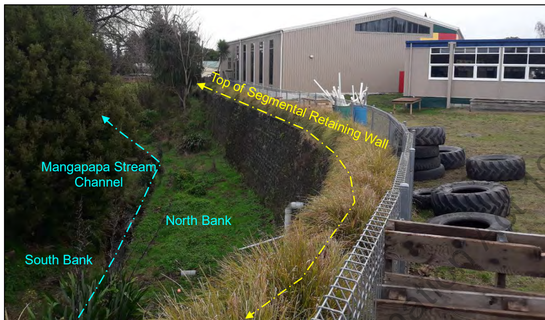
Figure 9: General view from top of segmental retaining wall facing south.
