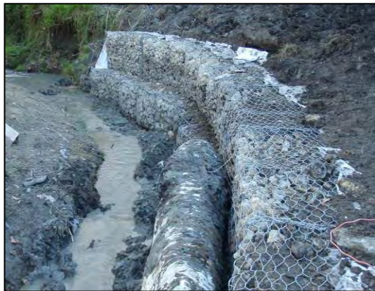
Figure 5f: 25/05/2012 – completed south gabions.
