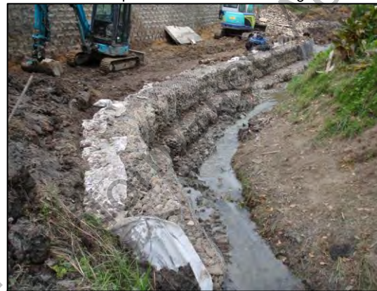
Figure 5g: 28/05/2012 – completed center and north gabions.
