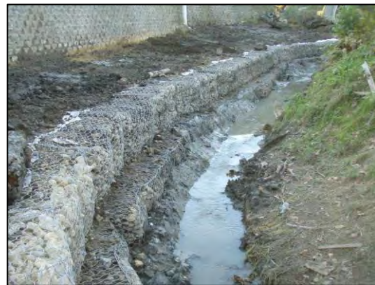
Figure 5i: 30/05/2012 – completed center and north gabions.
