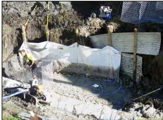
Figure 5d: 17/05/2012 – gabion in-construction.
