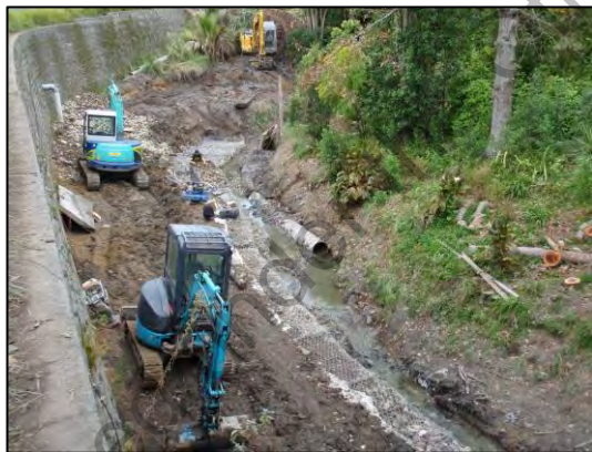
Figure 5h: 28/05/2012 – completed center and north gabions.
