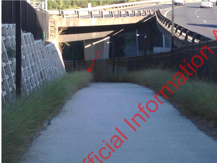
Figure 2: Encroaching grass obscures sight distance and narrows the path
