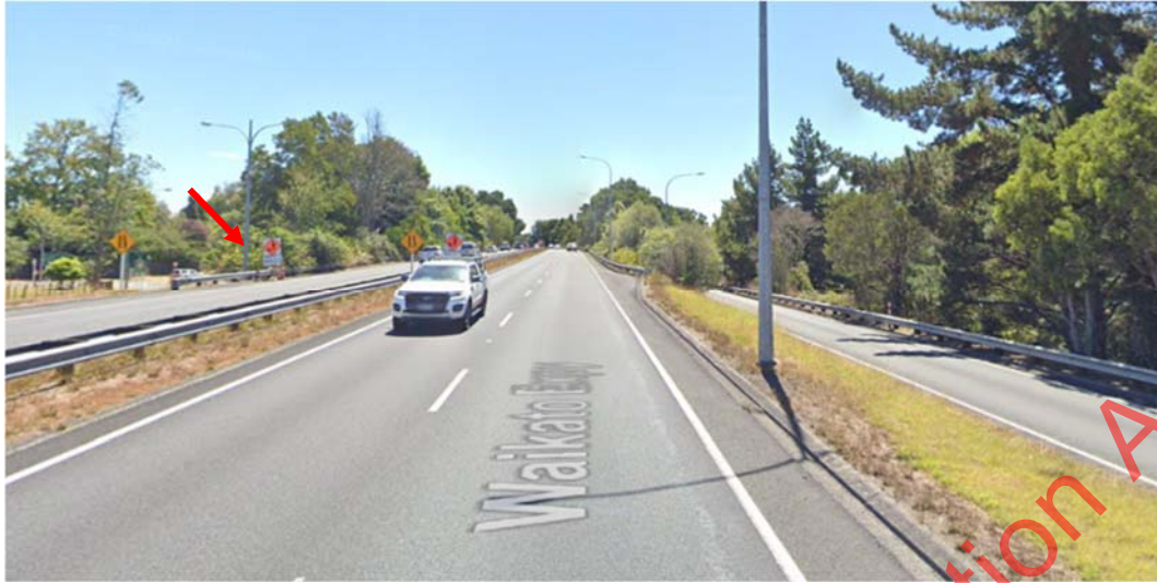
Figure 14: Lighting column close to edge of expressway (Google, 2021)
