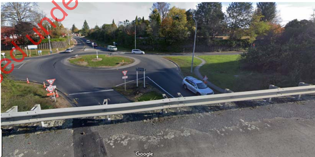
Figure 3: Bridge barrier (Google, 2021)
