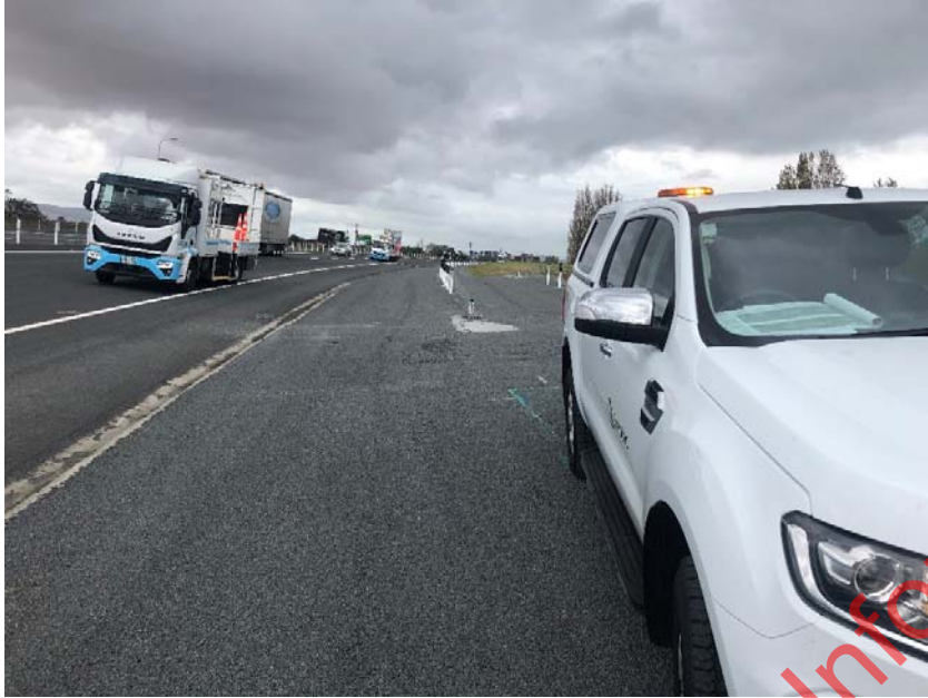
Figure 2: View from the maintenance bay break looking south.
