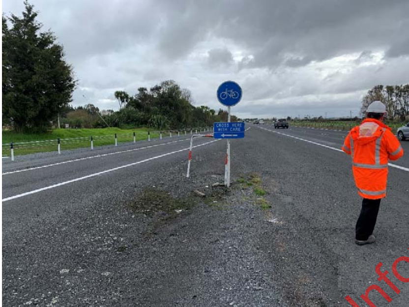
Figure 3: View looking south across Armitage Road On-ramp.
