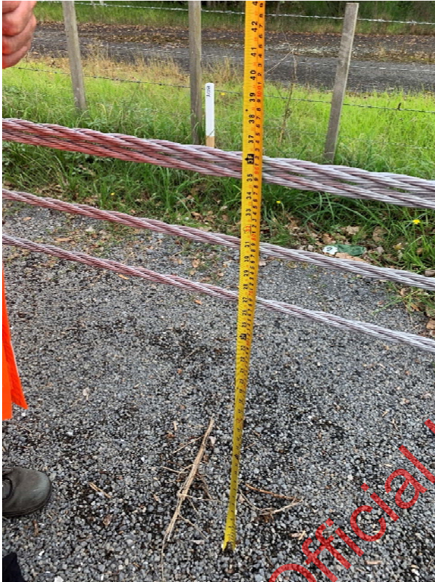
Figure 5: View depicting 680mm clearance under the bottom strand of wire
