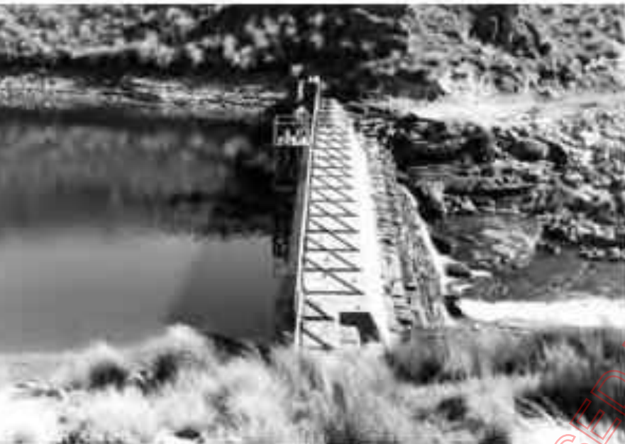
Figure 19. Lake Onslow Dam 1971
