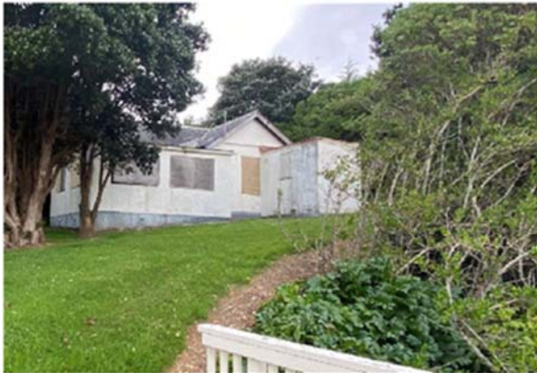
21 Bay Drive – Cable House
