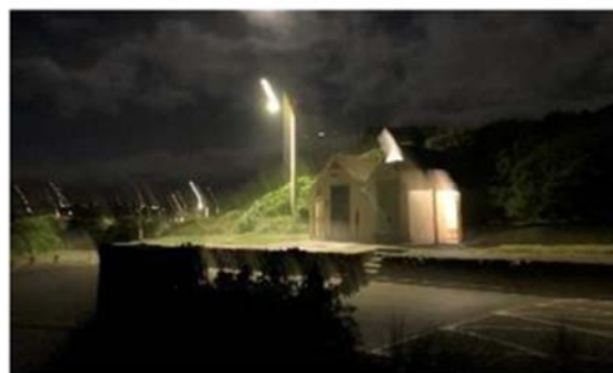
View of the public toilets from the parking
