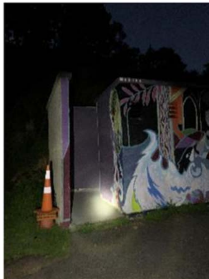
View of female toilet entry with powerful torchlight
