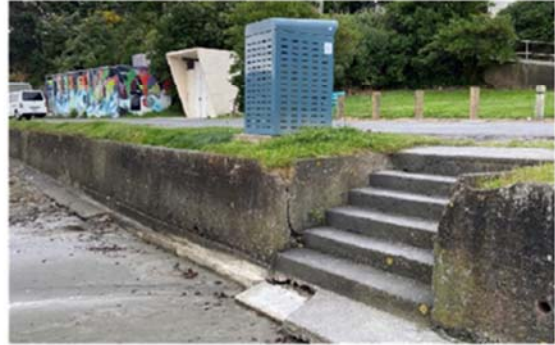
Sharp drop and broken steps - Vella Street
