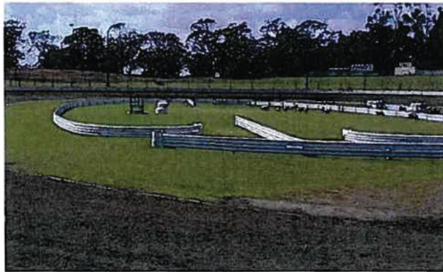
Fig. 6 View of barrier system in place on the infield at Borderline Speedway. Image taken from original provided by Tim Savell, CEO Speedway Australia.
