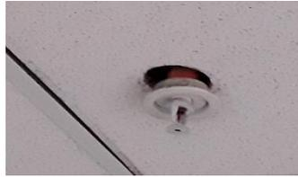
7. Room 315. Concealed sprinkler head dropped from ceiling. Contractor to confirm adequate pipework support. Refer photo below.
