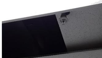
4. *Level 10. Common room. Ceiling tile lifted around sprinkler head. Refer photo below.*
