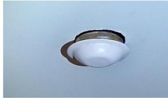
8. Room 218. Concealed sprinkler head dropped from ceiling. Contractor to confirm adequate pipework support. Refer photo below.
