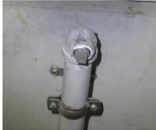
2. *Terrace Building, Level 7: The understairs sprinkler head is plugged off.*
