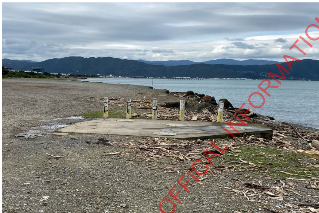
Figure 11: Gravel and debris creeps on existing path near KiwRail access track
