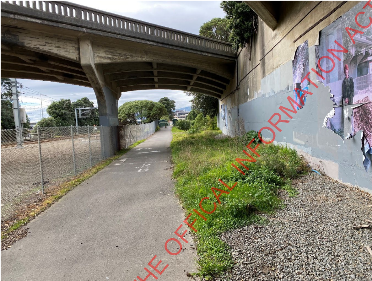
Figure 20: Existing intimidating environment below underpass
