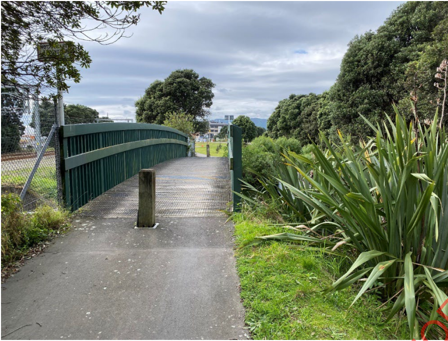
Figure 19: Existing pedestrian bridge within Honiana Te Puni reserve
