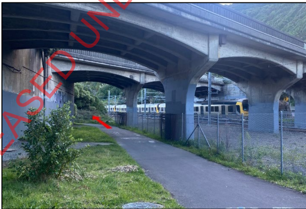
Figure 15: Petone interchange underpass, where the path will continue straight ahead
