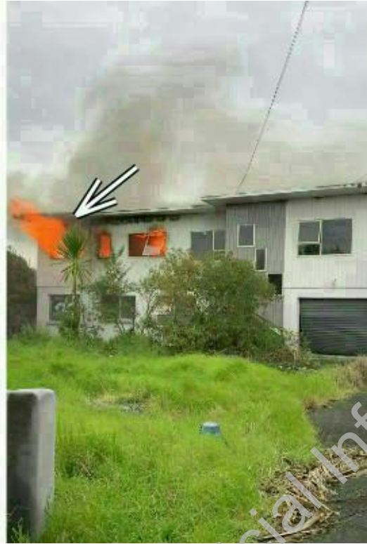
Image 2: Photo at the time of arrival of Manly DCFO. Arrow indicating area of origin.
