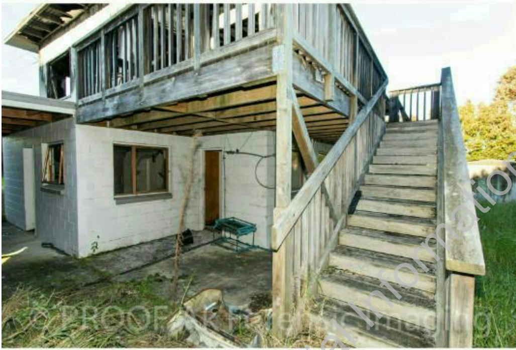
Photograph 15: Stairs leading to upper-level deck. (Courtesy of Police)
