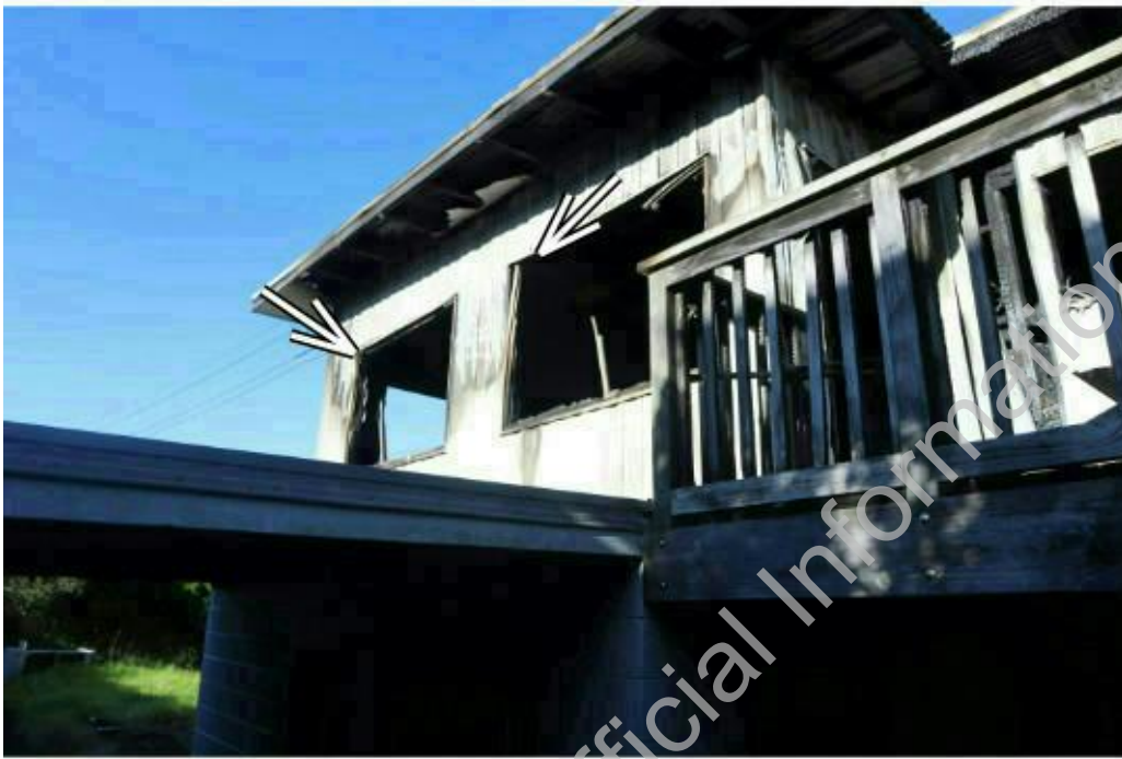
Photograph 10: Arrows indicating aluminium window frames on east profile.
