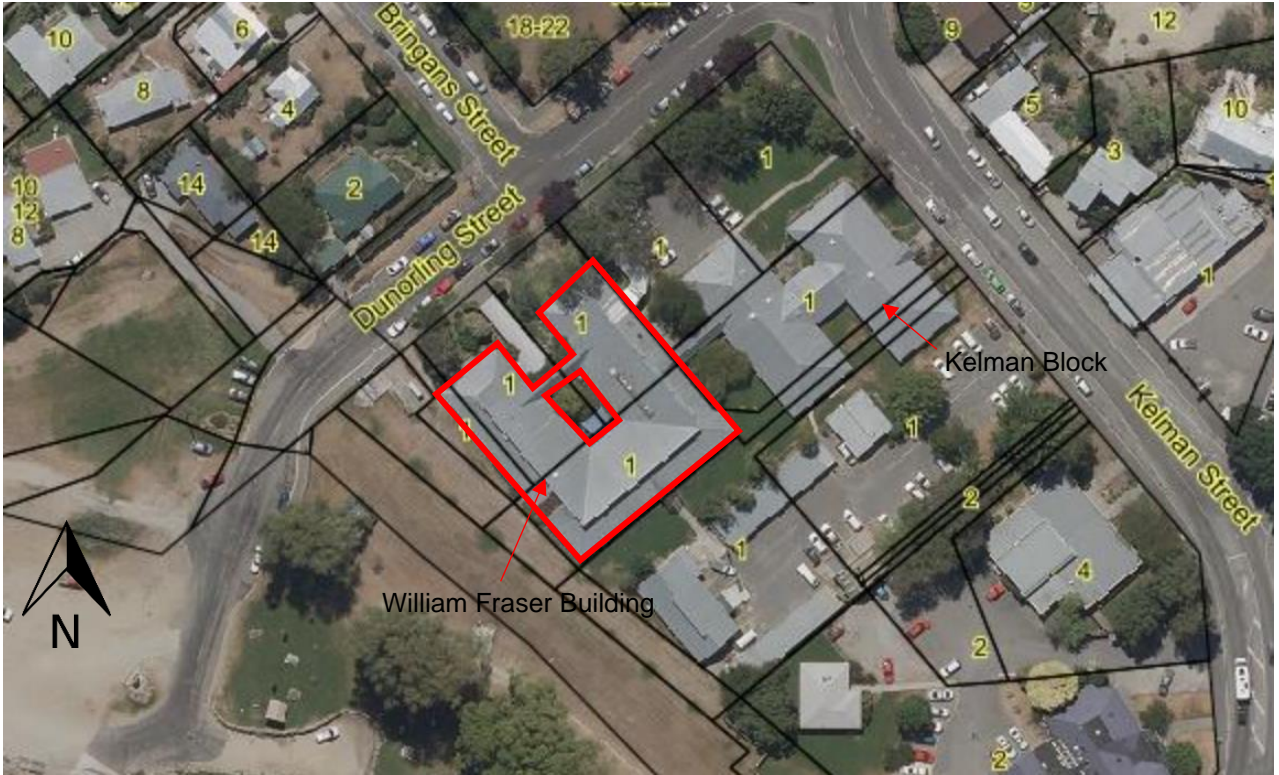
Figure 2: Aerial photograph of site (source: CODC GIS Maps)
