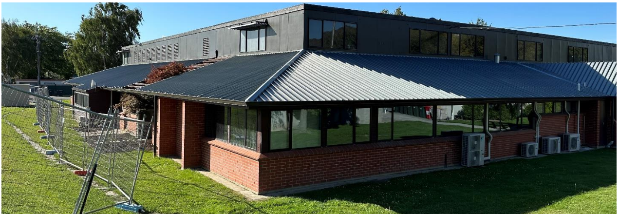
Figure 4: Rear view of William Fraser Block looking from the South direction.
