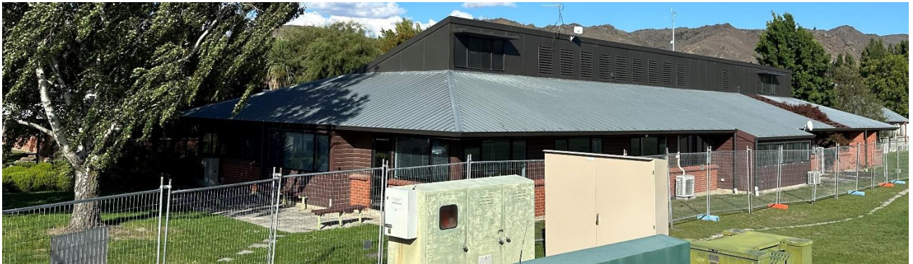
Figure 3: Front view of William Fraser Block looking from the West direction.
