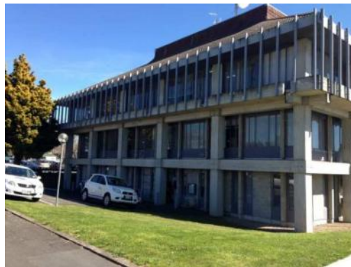
Figure 2.1 Photo of the Southeast Elevation showing the original structure with the basement level in-filled.
