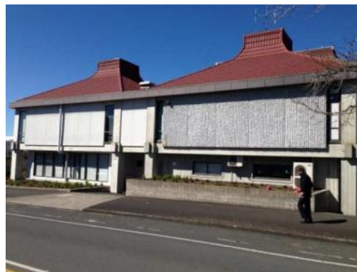
Figure 2.2 Northwest elevation showing original Council Chambers on the right and 1997 Alterations on the left.
