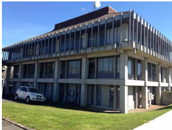
Figure 1 View of building from Roache Street
