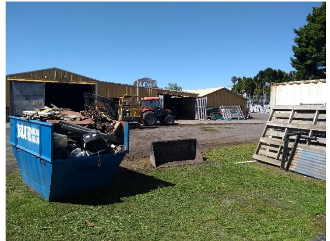
Figure 8 Storage at 2 Ash St, facing south.
