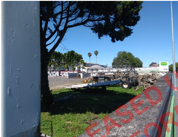
Figure 9 Machinery at 2 Ash St, facing west
