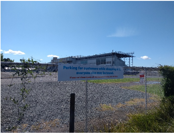
Figure 1 Northern portion of the site, facing south
