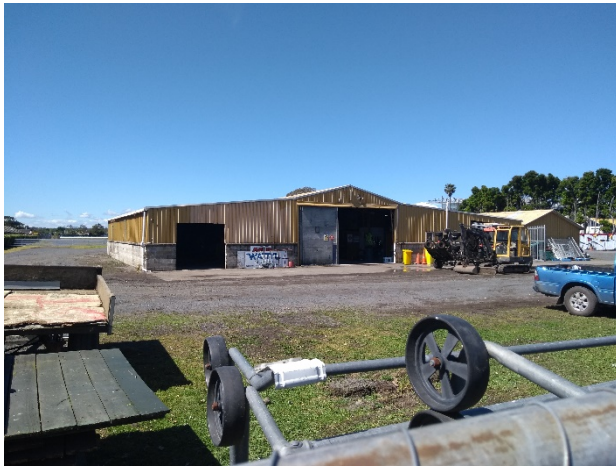
Figure 7 Warehouse at 2 Ash Street, facing south.
