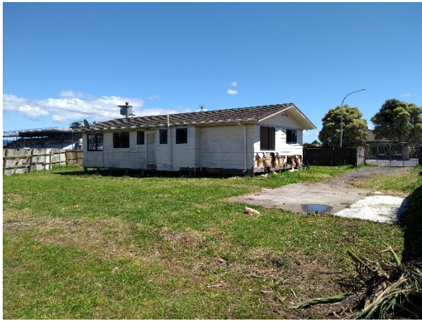
Figure 19 Dwelling at 22 Elm Street, facing north.
