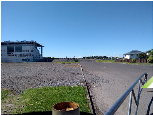
Figure 2 Northern portion of the site, facing south
