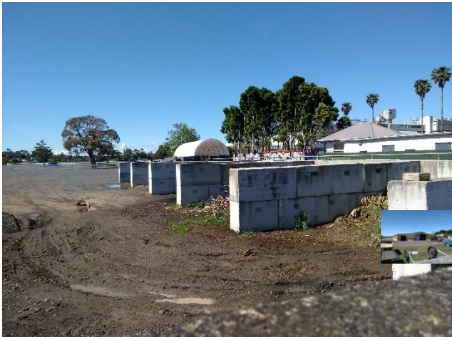
Figure 6 Equipment storage in north of site, facing southeast.
