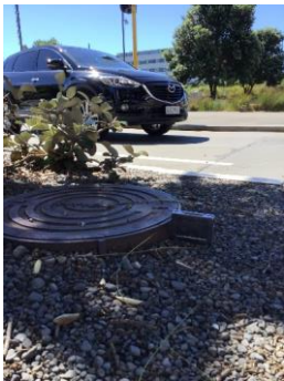
Figure 2-26: Service covers within proposed crossing point
