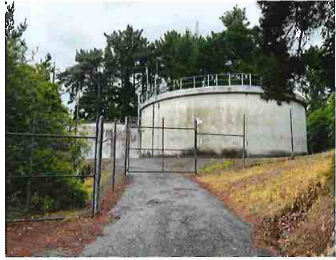
UHCC Water Supply Reservoir
