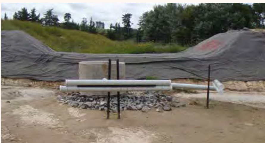
Sediment retention pond showing decant system.
