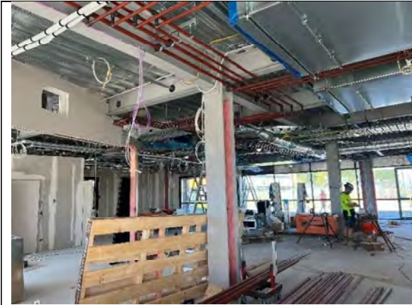
Photo 7 – View of Ground Floor Teaching Block
