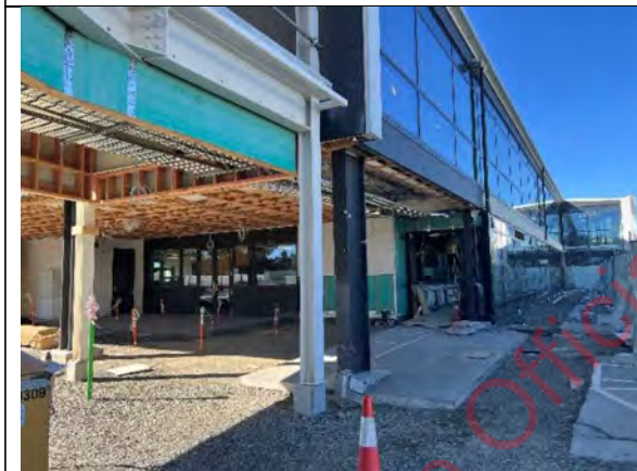
Photo 3 – View of Entrance to existing Tech Block
