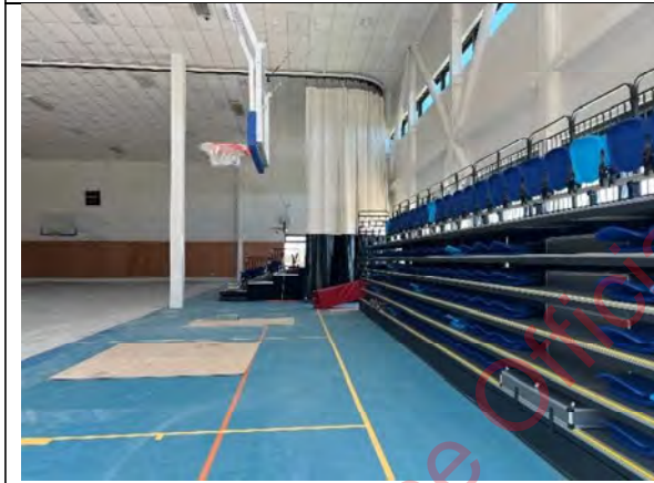
Photo 15 – Gymnasium existing floor
