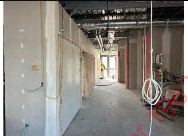
Photo 8 – View of Ground Floor Teaching Block
