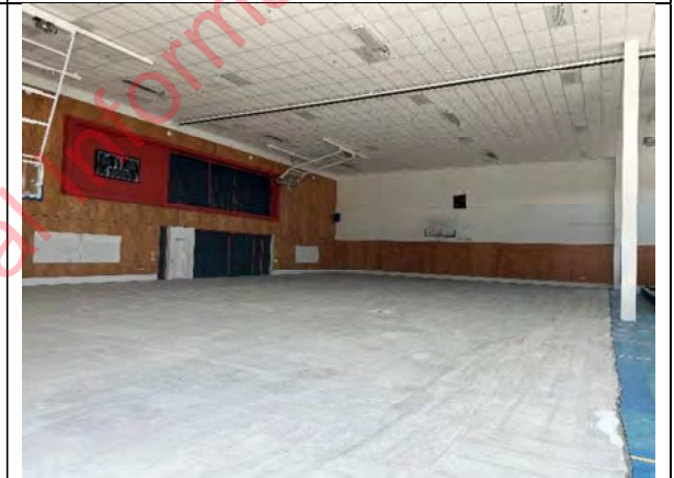
Photo 16 – Gymnasium old floor removed
