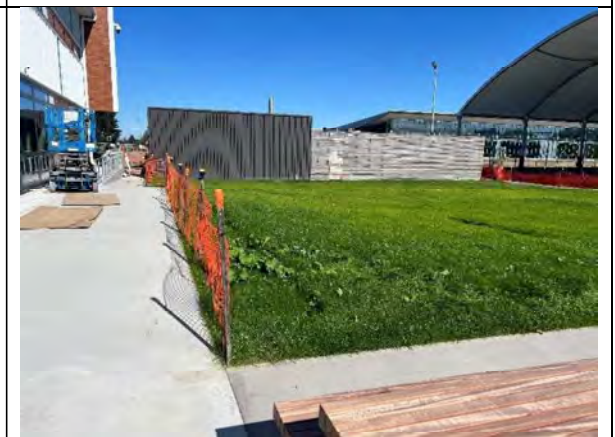
Photo 18 – Gymnasium landscaping progress
