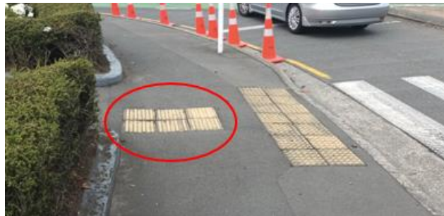
Figure 2-5: Incorrectly installed directional paving
