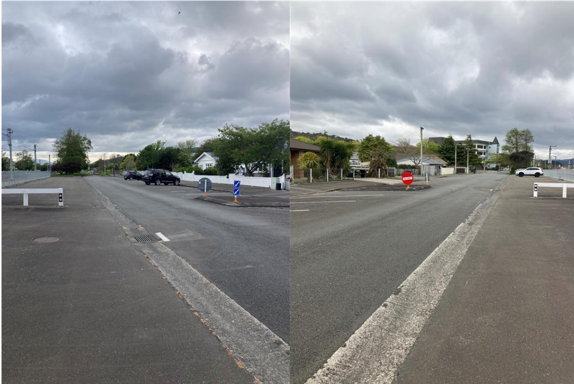
Figure 3.6 – Granville Road between Messines Avenue and Racecourse Road looking northwest (left hand side) and southeast (right hand side)
