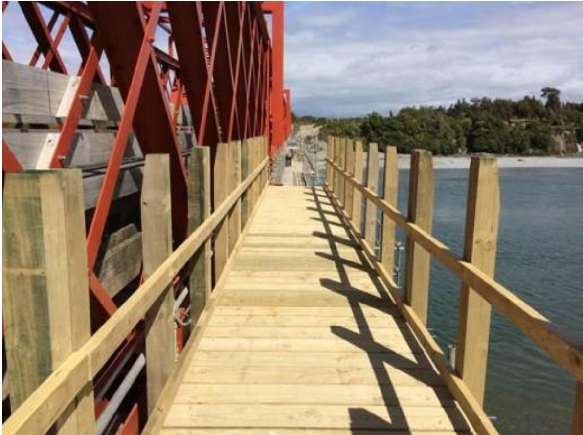
Figure 6 Taramakau Clip On Bridge (SH6) Under construction November 2015. Source NZTA
