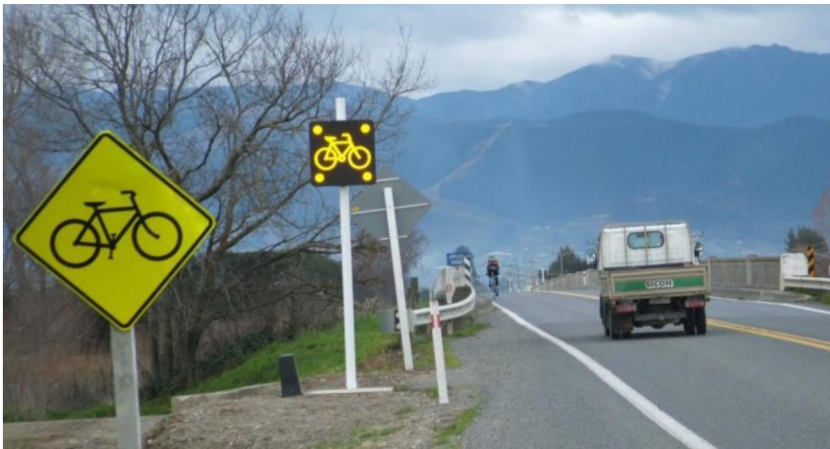
Figure 13 Inductive loop activated warning sign on narrow Appleby bridge, SH 60, near Nelson (NZTA/NZCT)
