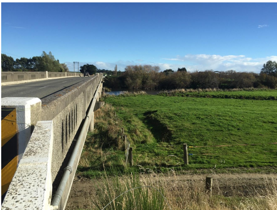
Figure 5 Mataura River Bridge showing potential position for clip-on bridge
