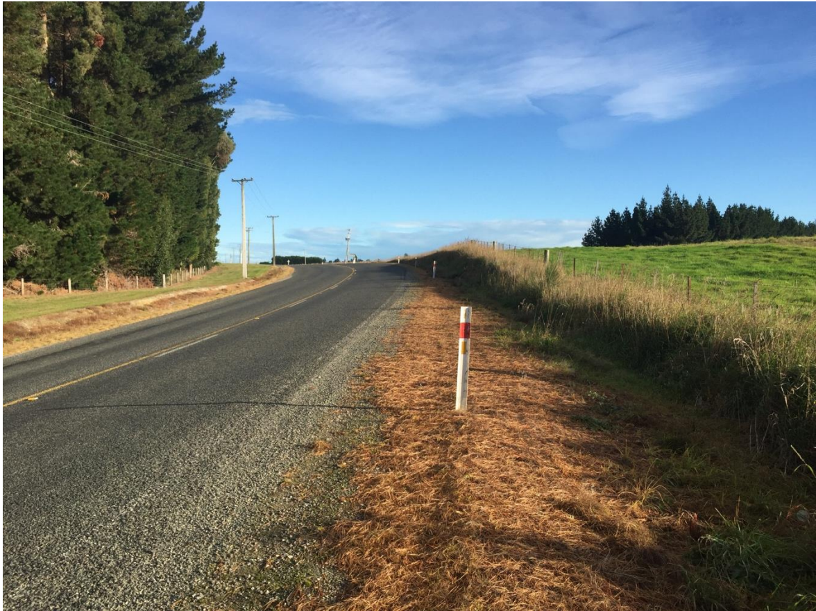
Figure 8 Edendale - Wyndham Rd Opposite Waste Water Treatment Plant
