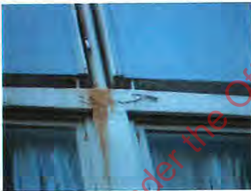
Rear Façade - Examples of Spalling Concrete
