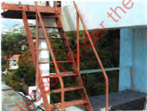
Access Stair to Lift Machine Room Badly Corroded
