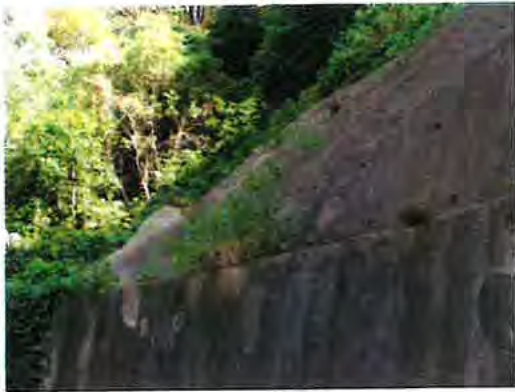
Sprayed Concrete Bank Greenery to be removed and Weep holes Cleaned
