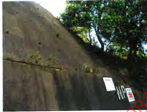
Sprayed Concrete Bank Greenery to be removed and Weep holes Cleaned
