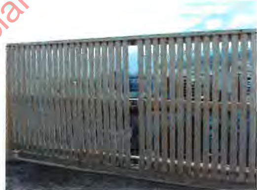
Palings missing from Security Fence
