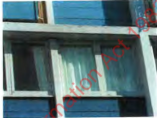
Minor rusting to Window Hinges.
