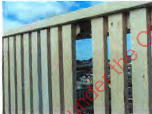
Palings missing from Security Fence
