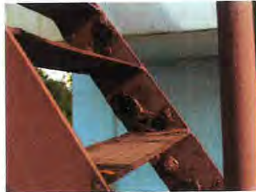
Access Stair to Lift Machine Room Badly Corroded
