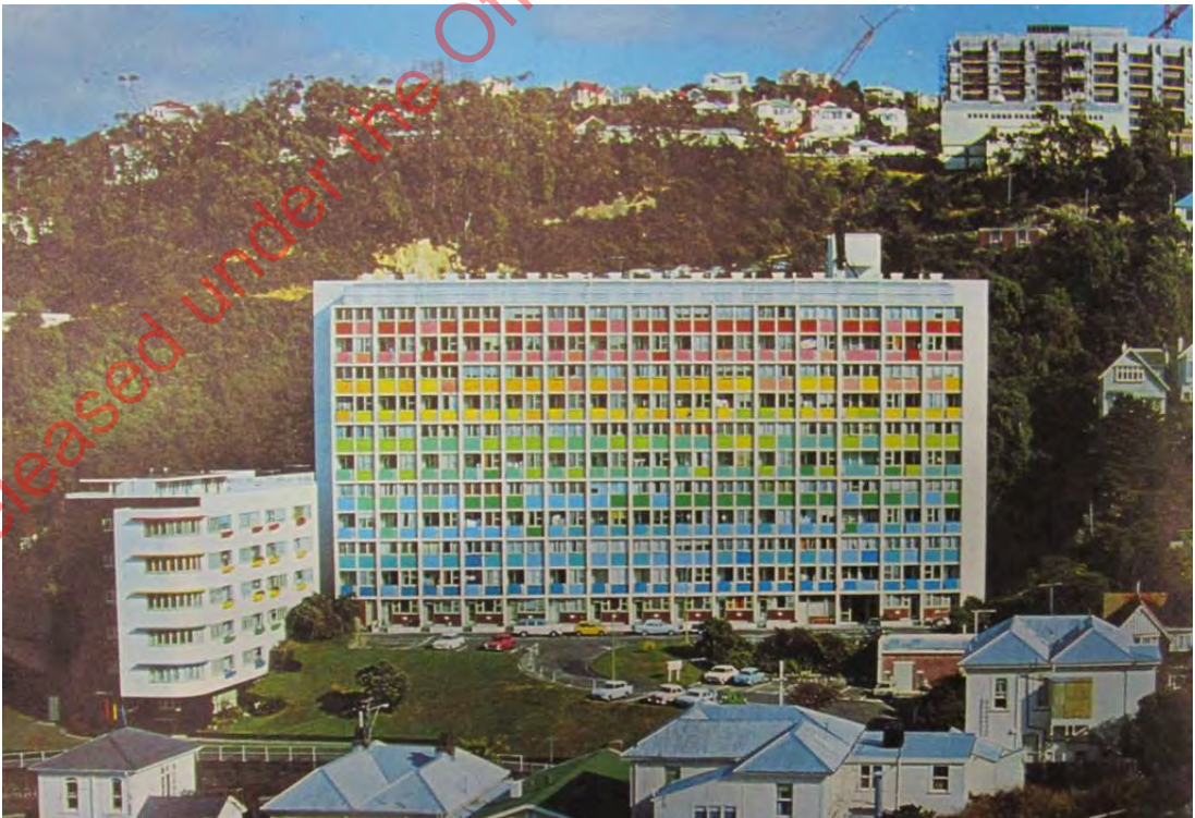
Figure 8: Gordon Wilson Flats, and the Mclean Flats, had a multi-coloured paint scheme in the late 1970s, inspired by a Dulux paint chart (pers comm. Chris Cochran, a colleague in the MOW office at the time, to Heritage New Zealand 3 September 2020). The image is reproduced from New Zealand Architect , issue no 5 1978, p. 29
