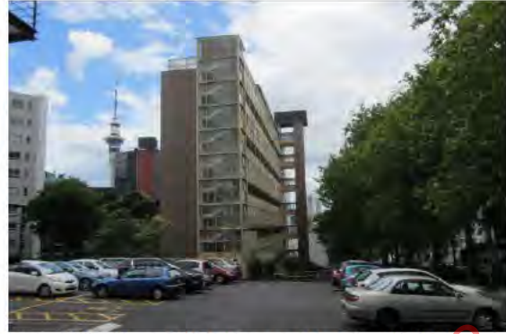
Figure 86. View of flats from neighbouring YMCA hostel. (Archifact-Architecture & Conservation Ltd., 2014)
