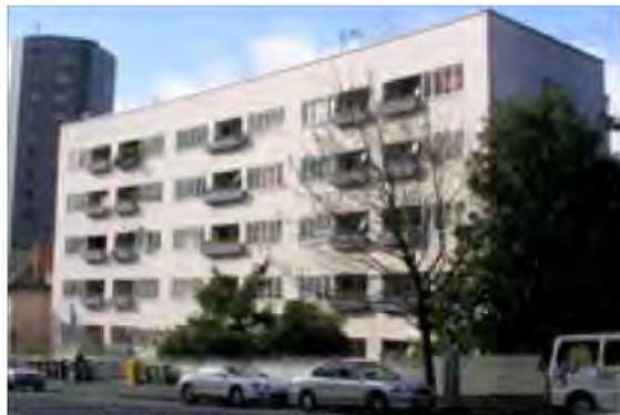
Figure 77. Street view of flats, showing colour scheme.
