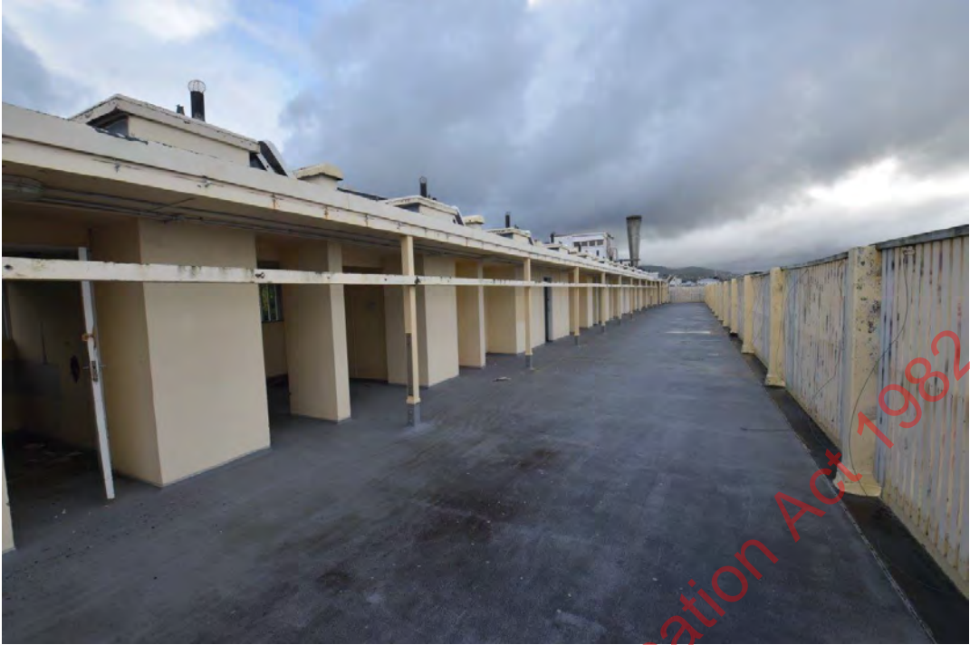
Figure 13: Gordon Wilson Flats' rooftop laundry facilities.
