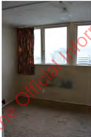
Figure 57. Looking at a typical east side bedroom. Note damp patch with mould growth on the external wall. (Archifact-Architecture & Conservation Ltd., 2014)
