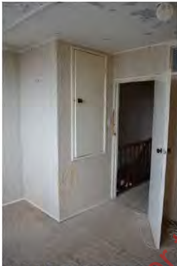
Figure 56. Looking at a typical east side bedroom. (Archifact-Architecture & Conservation Ltd., 2014)
