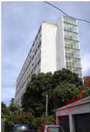
Figure 18. Looking at the north end of the building with the glazed access stairwell set on the north-east corner of the building. (Archifactor-Architecture & Conservation Ltd., 2014)
