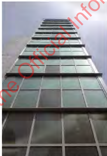
Figure 19. Looking up at the glazed elevation of the northern stairwell. (Archifactor-Architecture & Conservation Ltd., 2014)
