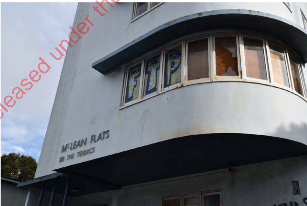
Figure 10: Detail of east elevation of McLean Flats.
