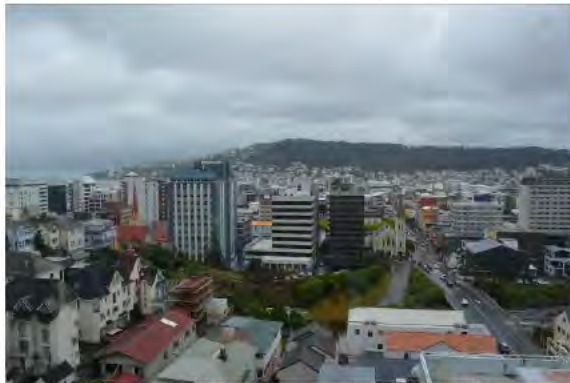
Figure 61. A typical view from an apartment looking towards the east. (Archifact-Architecture & Conservation Ltd., 2014)
