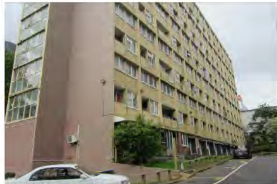
Figure 90. Rear façade of flats. (Archifact-Architecture & Conservation Ltd., 2014)
