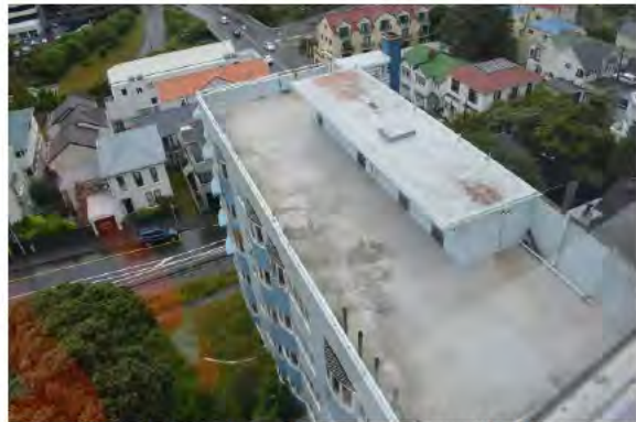
Figure 62. A typical view from an apartment looking towards the McLean Flats which are situated at the southern end of the site. (Archifact-Architecture & Conservation Ltd., 2014)
