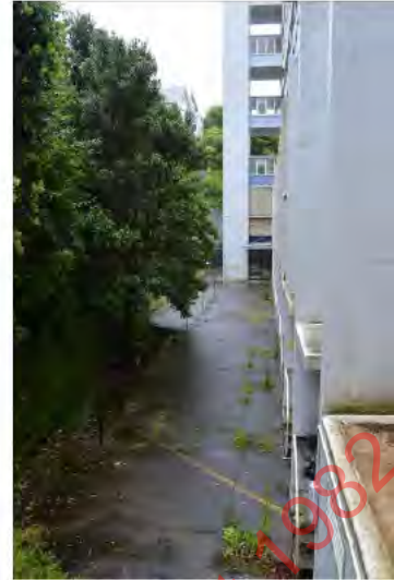
Figure 23. Looking north along the western elevation. Note the slender buttresses on the right of the image that act as stiffening members anchoring the structure to the pile heads. (Archifact-Architecture & Conservation Ltd., 2014)
