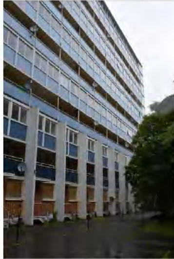
Figure 22. Looking south along the western elevation. Note the slender buttresses that act as stiffening members anchoring the structure to the pile heads. (Archifact-Architecture & Conservation Ltd., 2014)
