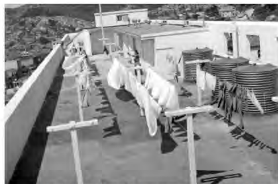
Figure 76. Rooftop laundry rooms, similar to those found on the Gordon Wilson Flats. (Source: Part of the roof of the Dixon Street Flats, Wellington. Pascoe, John Dobree, 1908-1972 :Photographic albums, prints and negatives. Ref: 1/4-000820-F. Alexander Turnbull Library, Wellington, New Zealand. http://natlib.govt.nz/records/23066090 )
