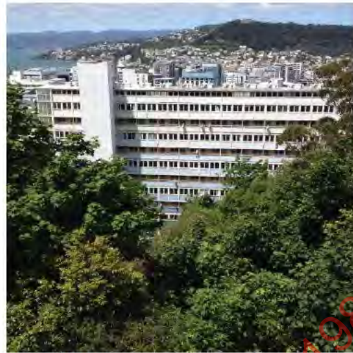
Figure 17. Looking west towards the Gordon Wilson building with the city context in the background. (Archifact-Architecture & Conservation Ltd., 2014)
