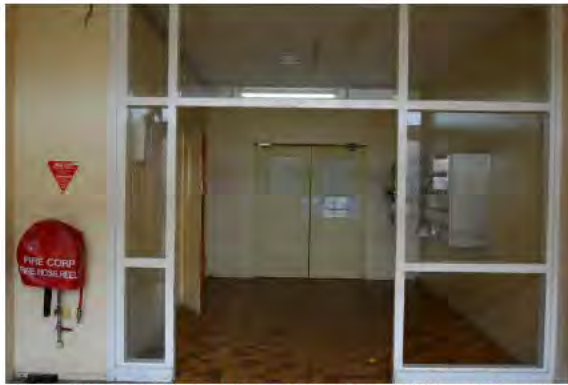
Figure 38. Looking at the main entrance lobby at Ground Floor level. (Archifac-Architecture & Conservation Ltd., 2014)
