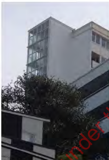
Figure 24. Looking at the upper levels of the southern end of the building with the glazed access stairwell set onto the south-west corner of the building. (Archifact-Architecture & Conservation Ltd., 2014)
