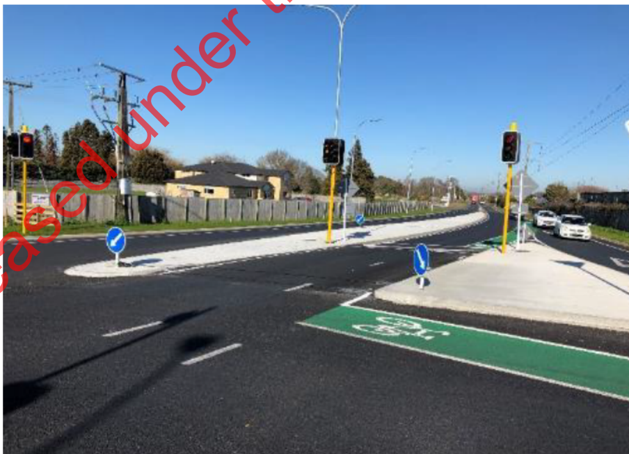
Figure 2: Raised safety platform (northbound lane)
