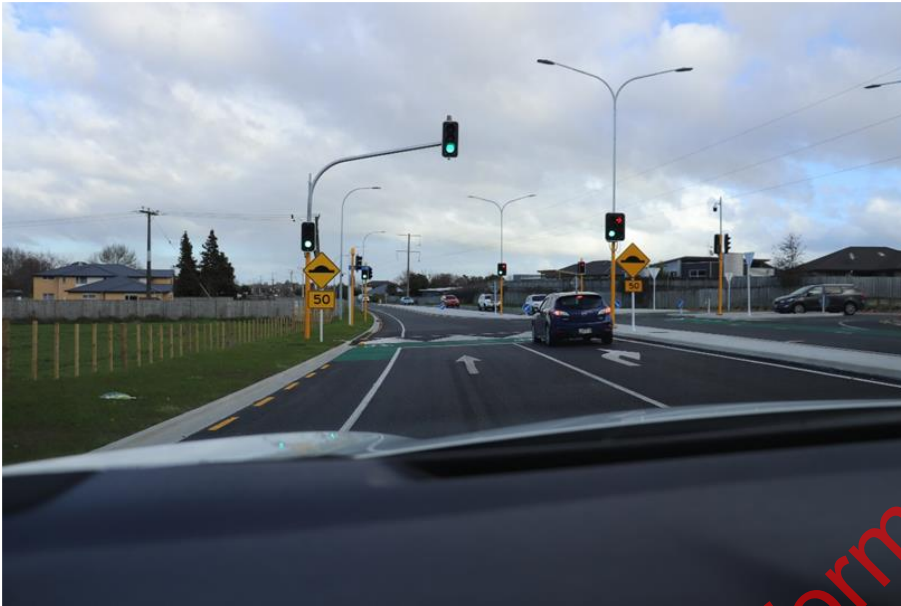
Figure 6 shows the northbound view exiting the intersection and the speed threshold transitioning from the 60km/h to 80km/h speed limit.
