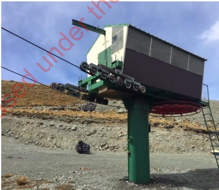
Figure 2 – T Bar Drive Station
