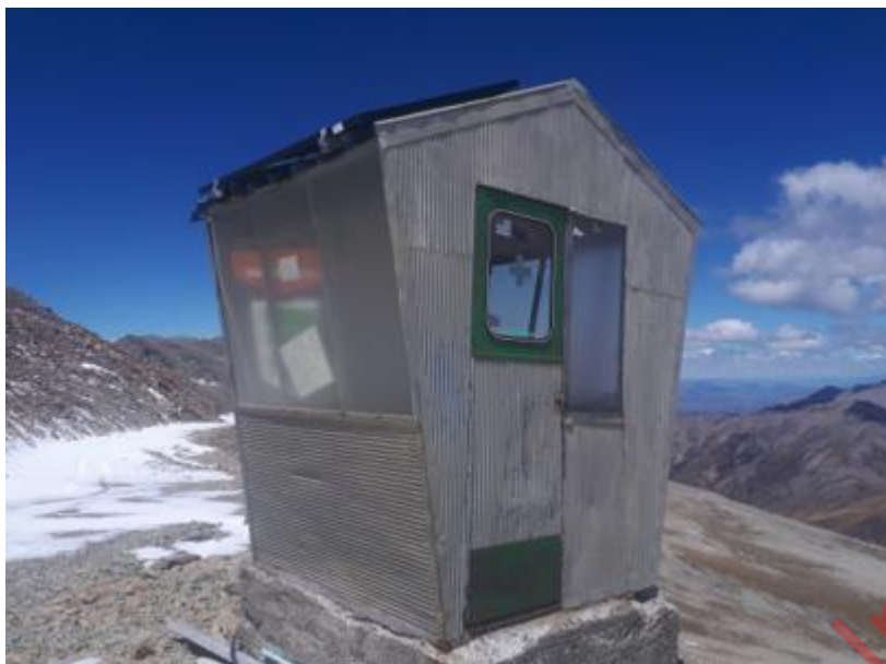
Figure 11 – Top of the T Bar Operators Hut
