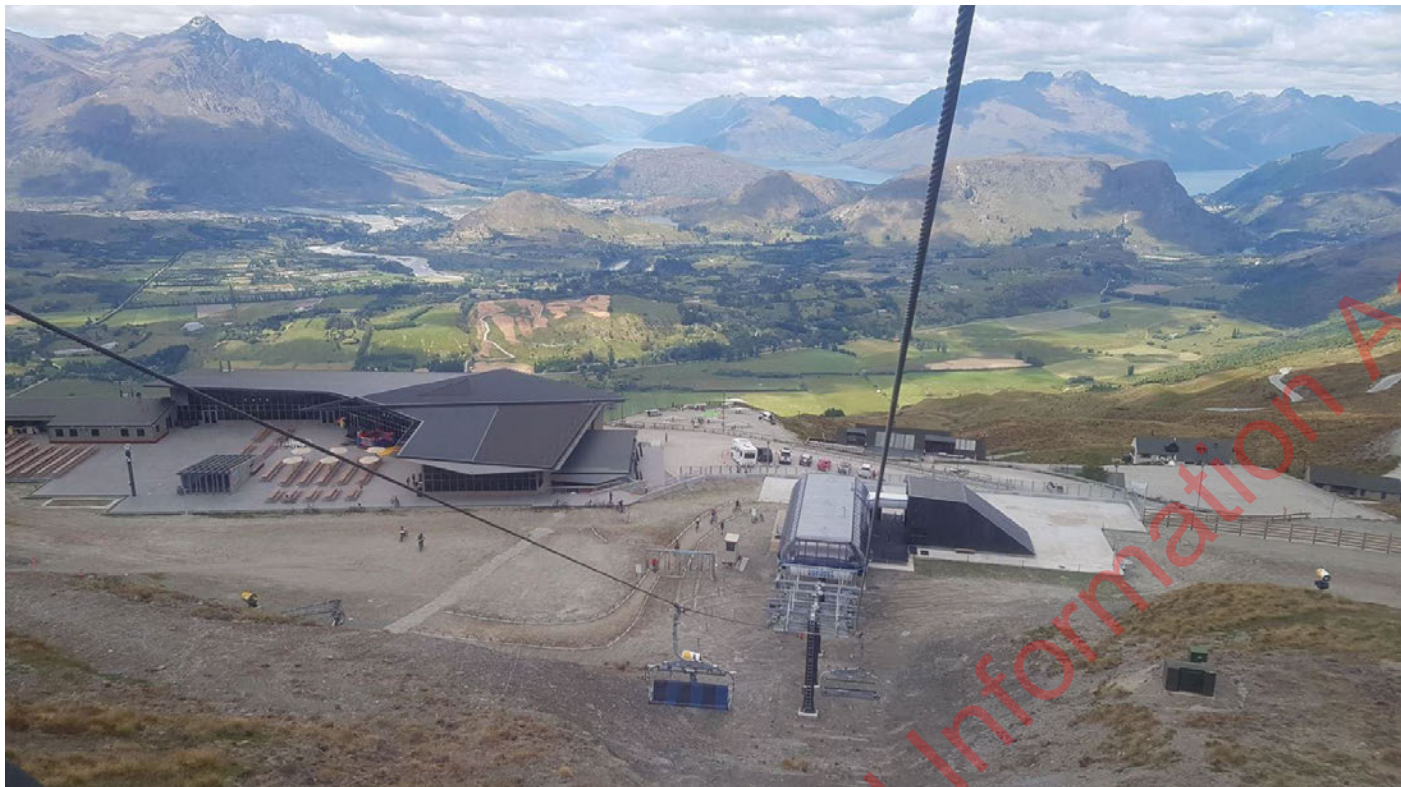
Figure 4.3(b): View looking down from the Coronet Express return top station towards the completed drive bottom station, service building and parking garage
