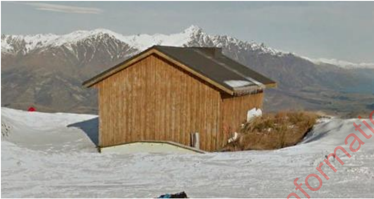
Figure 21: PS400 Big Easy Pump Shed & Bore - 38m 2
