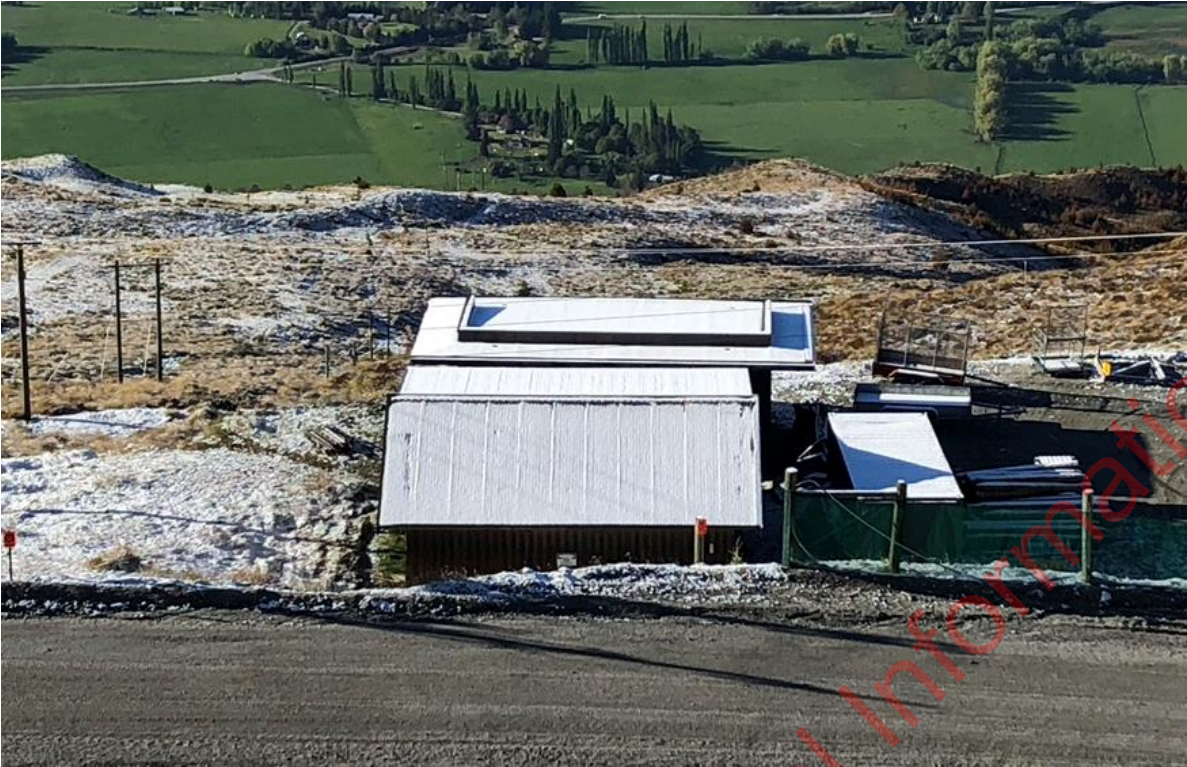
Figure 27: Power Factor Hut - 102m 2
