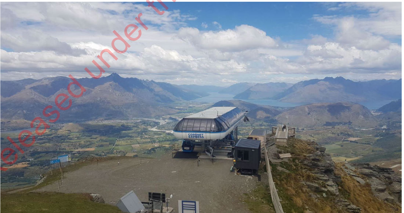
Figure 4.3(a): Completed replacement of Coronet Express return top station and service building. Gondola cabin can be seen attached to chairlift on left hand side
